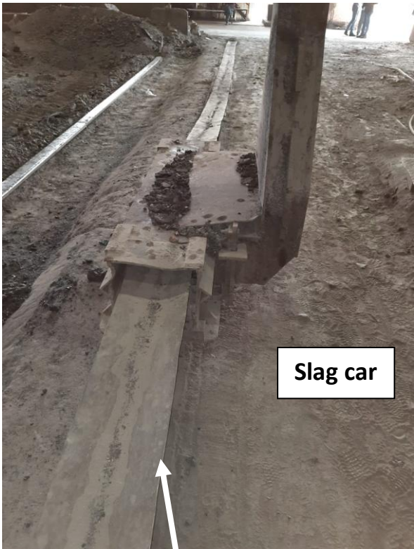
Thin metal strip is provided over the opening of trench of underground bus bar to protect from entering of foreign material.
